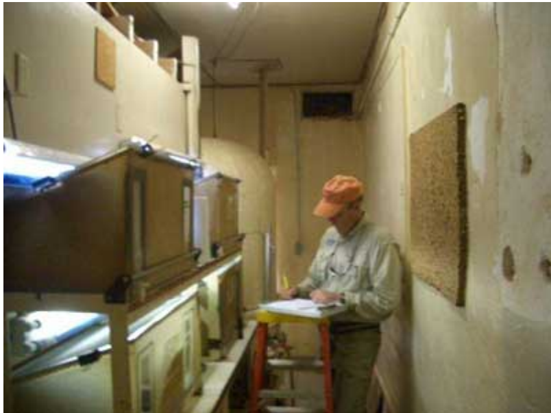
Robert Breen of EFS completes "As Built's" on the Mountain House
